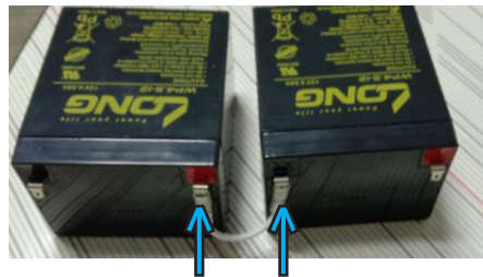
Replace New Batteries and Plug In Terminal Into New Batteries
