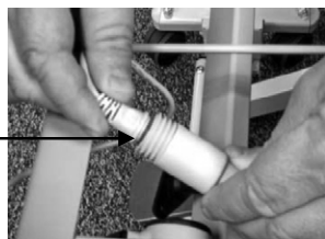
Improper Connection (not completely seated)
